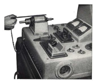
Fig. 325 - Testing the armature on bench, using a lamina. In correspondence with short-circuited coils the lamina will vibrate.
