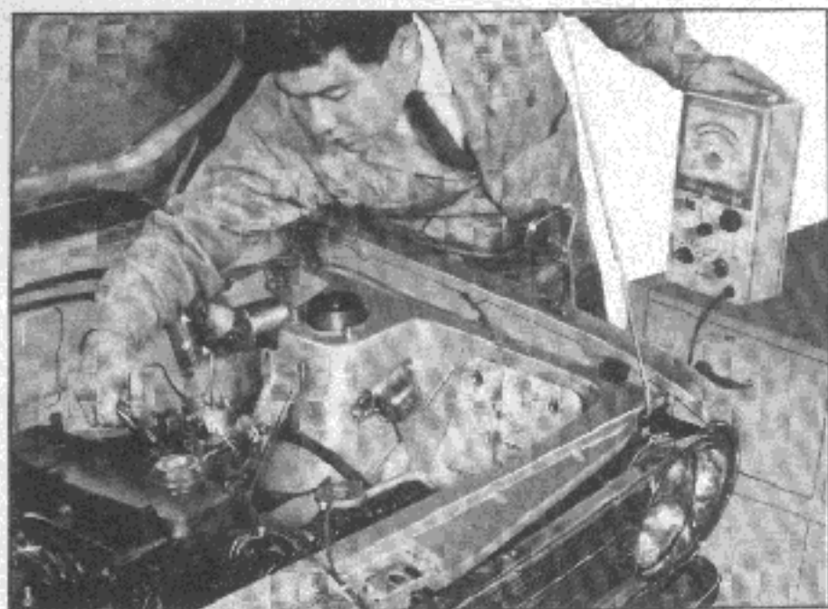
Fig. ET-7 Idle adjustment
