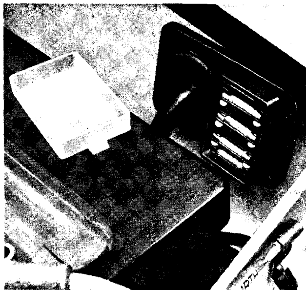
Fig. 3. Fuse assembly installed
