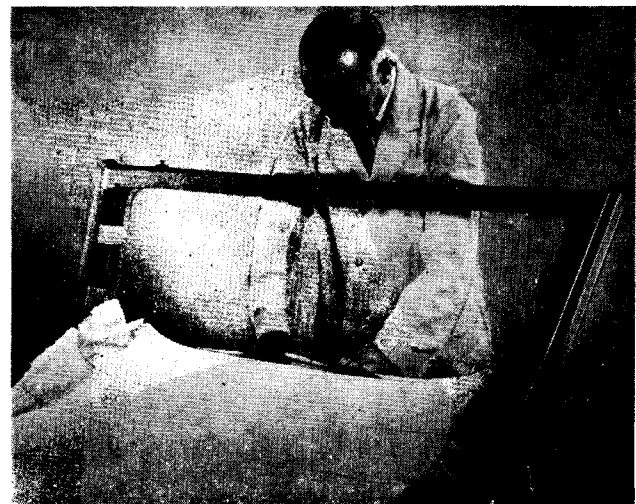
Fig. 50. Securing rear edge of roof lining
