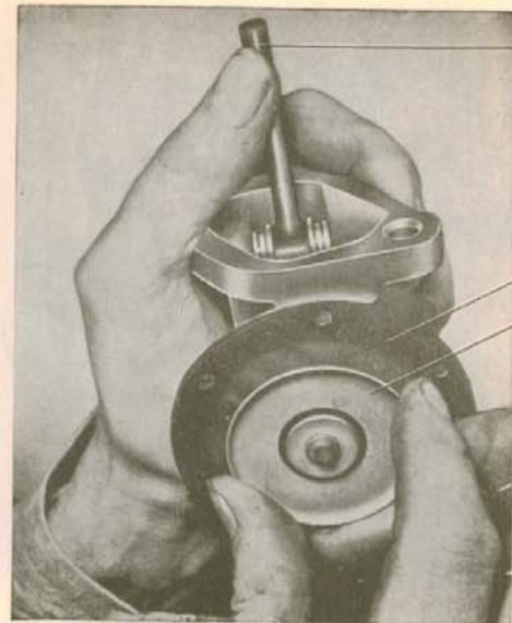
Fig. 1-81. Replacing the diaphragm
