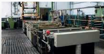
Phosphate coating plant
